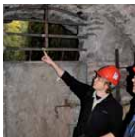
Survey of tunnel owned by Bristol Water, to check on access created for hibernating bats.
